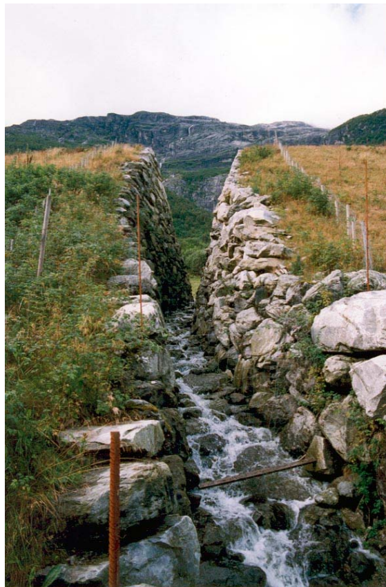
Photo no 11. Detail of the opening in the catching dam
