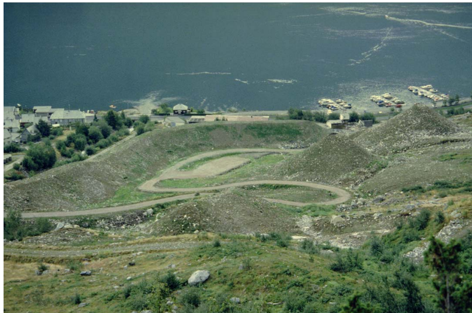
Photo no 7. View of the mitigations at Egne Hjem securing the housing area and the road against avalanches
