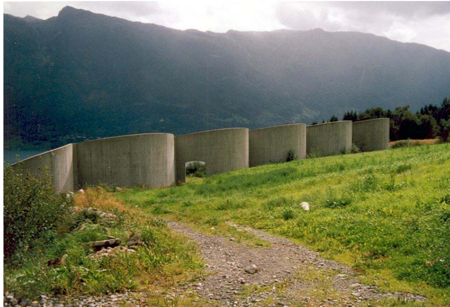
Photo no 9. View of the catching wall at Reiseter
