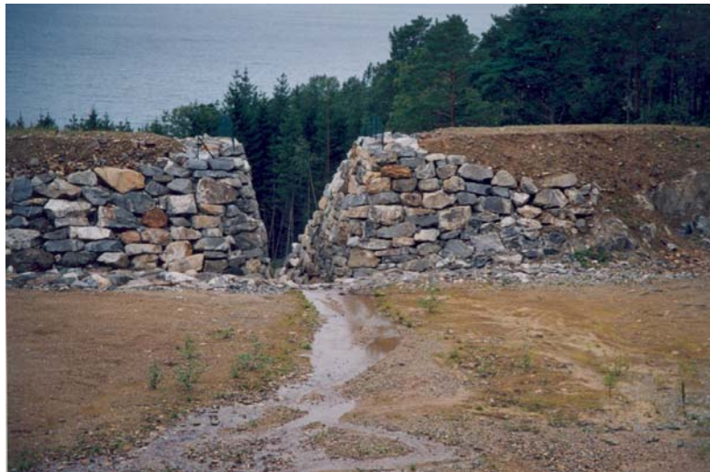
Photo no 5. In the lower part of the channel area a wider accumulation basin is built, with an opening in the middle to allow water drainage. This also permits accumulated masses to be eroded out of the accumulation area. We expect some maintenance after each debris flow. A road over the dam permits access to the channel area for maintenance.
