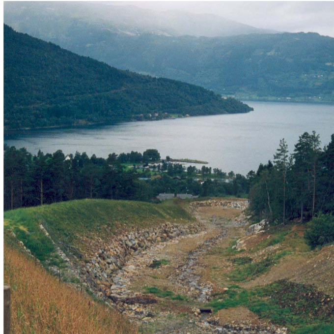
Photo no 4. A 5 m – 10 m high channel dam was built to prevent housing areas in the central part of Kinsarvik to be hit by debris flows.
